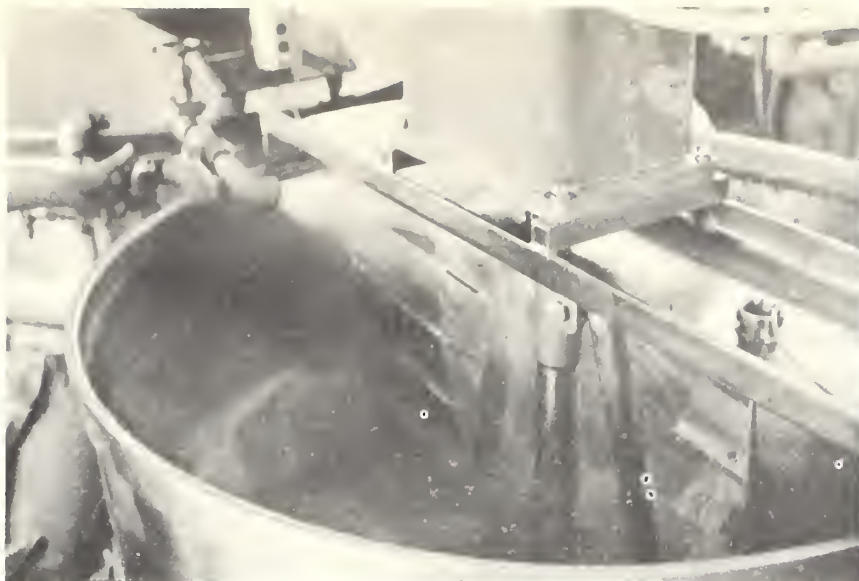
Figure 9.--A 600-pound batch of Redi Wheat is cooked in a steam-jacketed kettle with continuous stirring.
